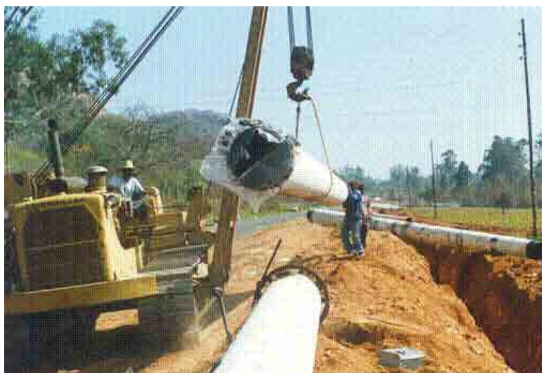
Figure 14: Trench and working area for pipe lying
